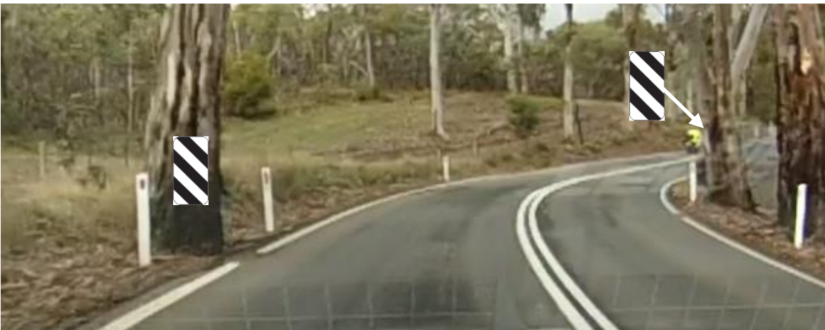
Figure 4.30: Hazard sign on trees in shoulder
