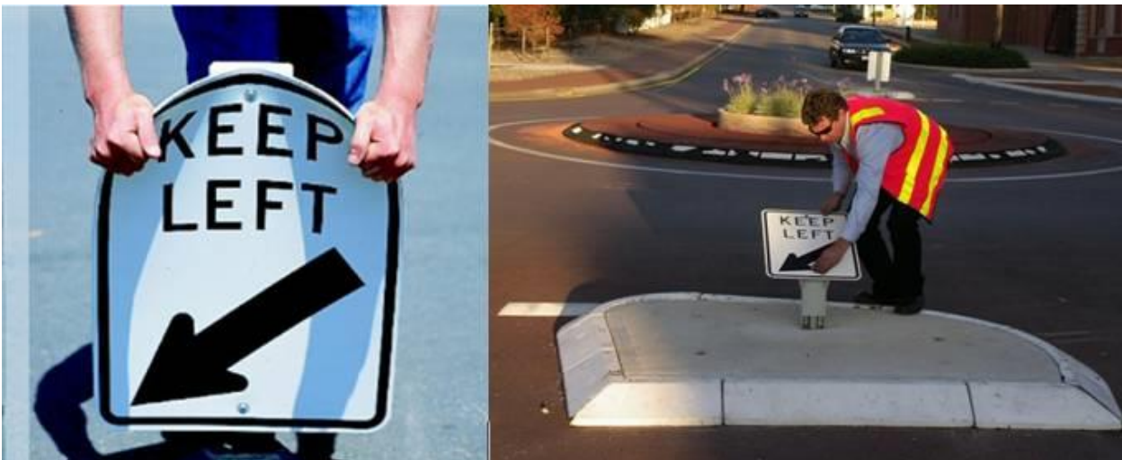
Figure 5.12: Flexible intersection sign posts and sign faces (keep left sign)
