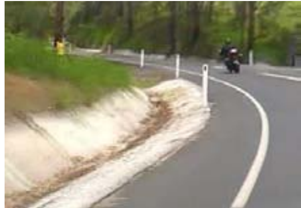
Traversable drainage treatment
