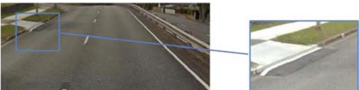
Figure 4.64: Driveway kerbing in shoulder
