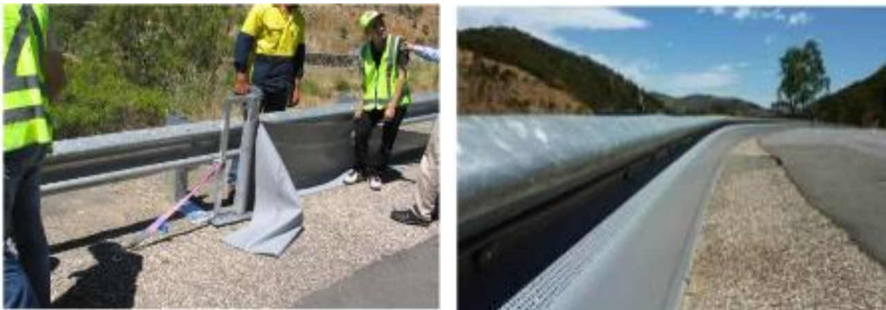
Figure 2.5: Installation and view of the flexible barrier protection system (see Section 1.4)
