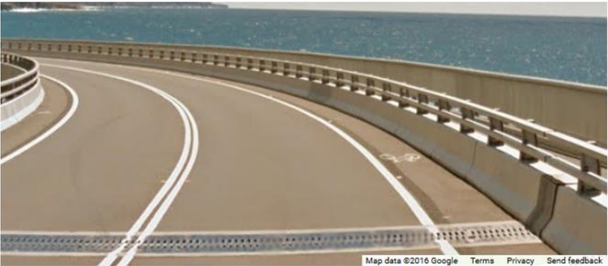
Figure 4.57: Bridge join on a curve
