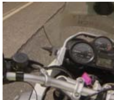
Longitudinal cracking on concrete slabs
