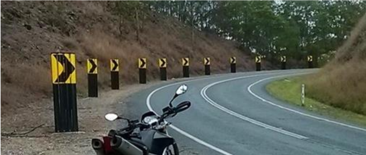
Figure 5.9: Flexible chevron alignment markers
