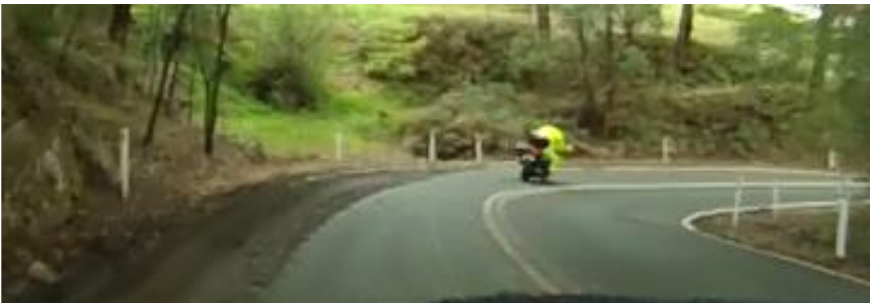
Figure 4.55: Debris from shoulder on curve
