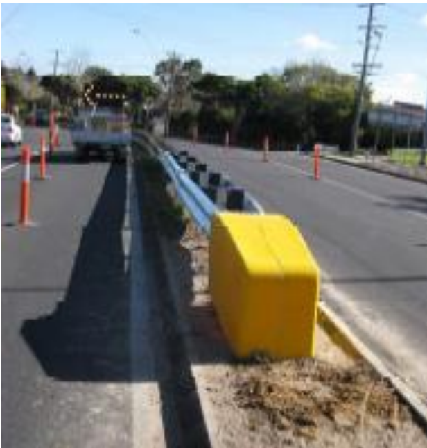
Figure 5.17: Guardrail – X350 cover over sharp edges
