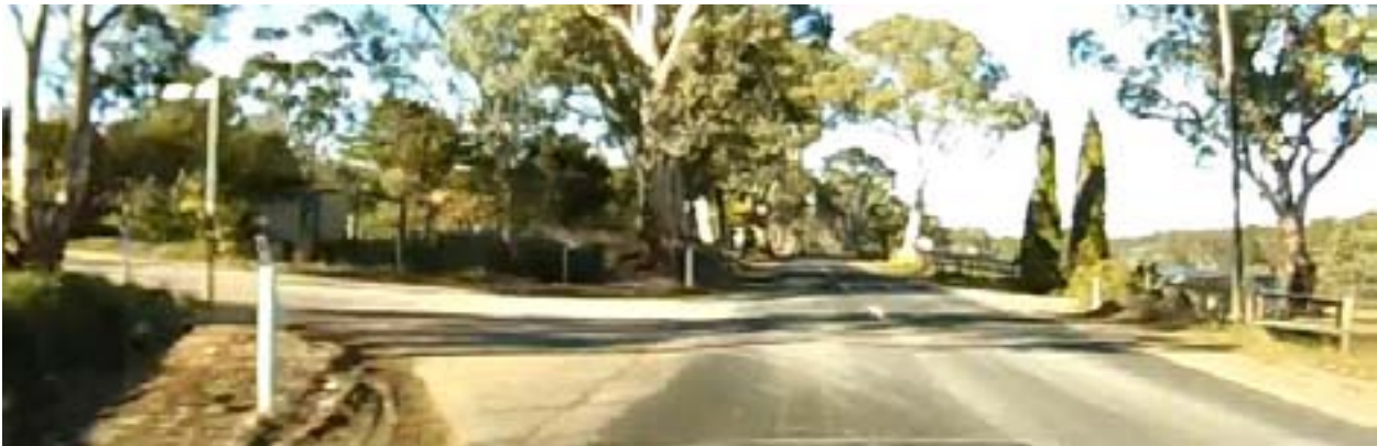
Figure 4.54: Debris on road from unsealed side road
