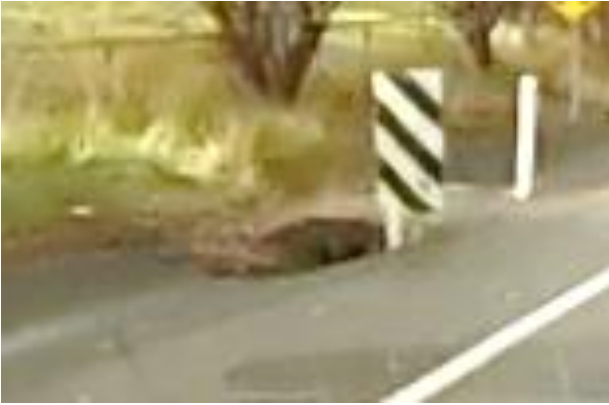
Figure 4.118: Culvert end wall and gully pit wall perpendicular to through road
