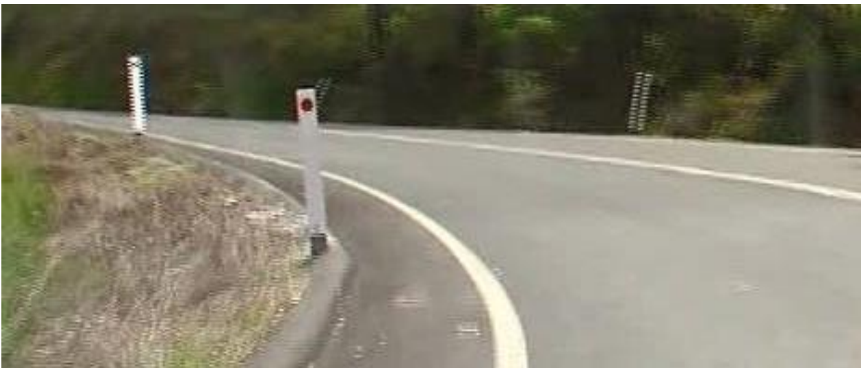
Figure 4.63: Cold mix kerbing, not conspicuous
