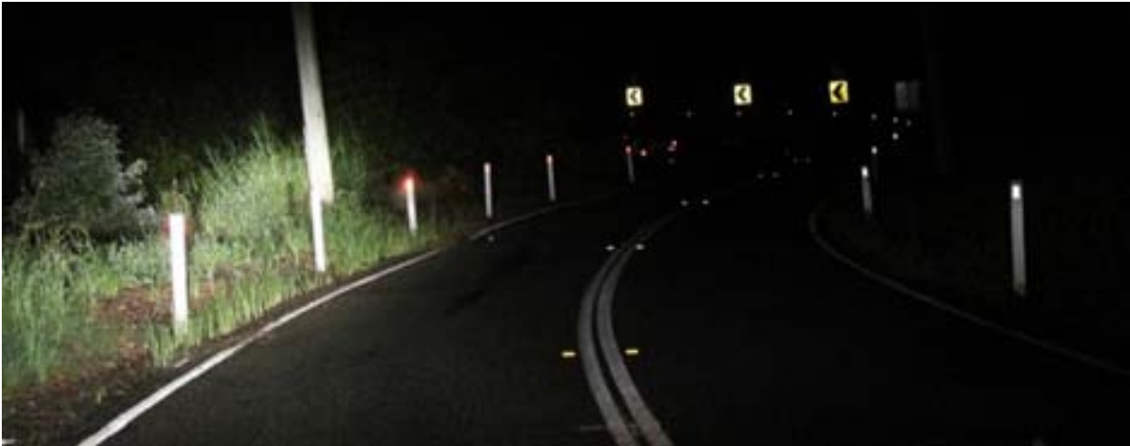
Figure 4.40: Curve quality at night, guide posts at closer spacing on a reverse curve
