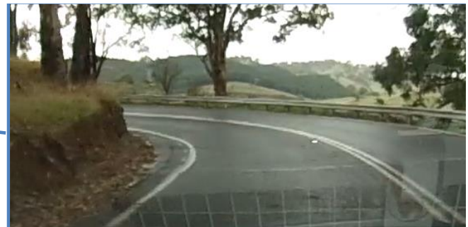
Figure 4.41: CAMs not provided on reverse compound curve with sharp curve warning and speed advisory plate
