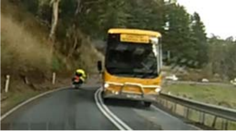
Figure 4.24: Narrow lane and shoulder width
