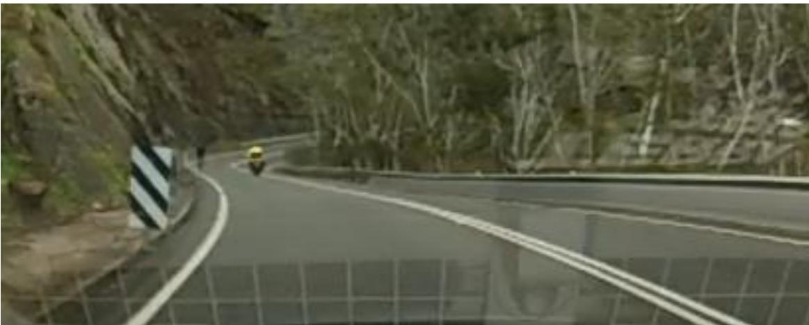
Figure 4.31: Hazard sign on drainage ditch
