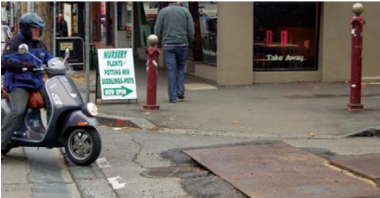
Figure 4.60: Steel plates over trenches
