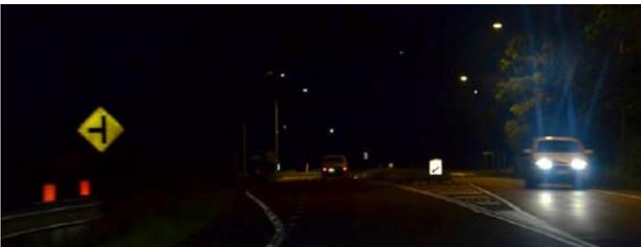
Figure 4.95: Poor lighting and delineation left turn lane and centre median crossing
