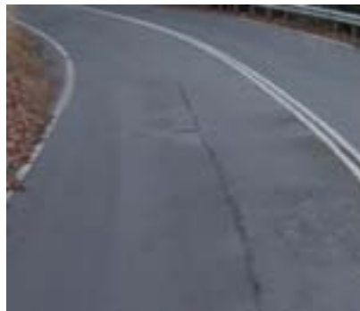
Pavement repair construction joint on curve
