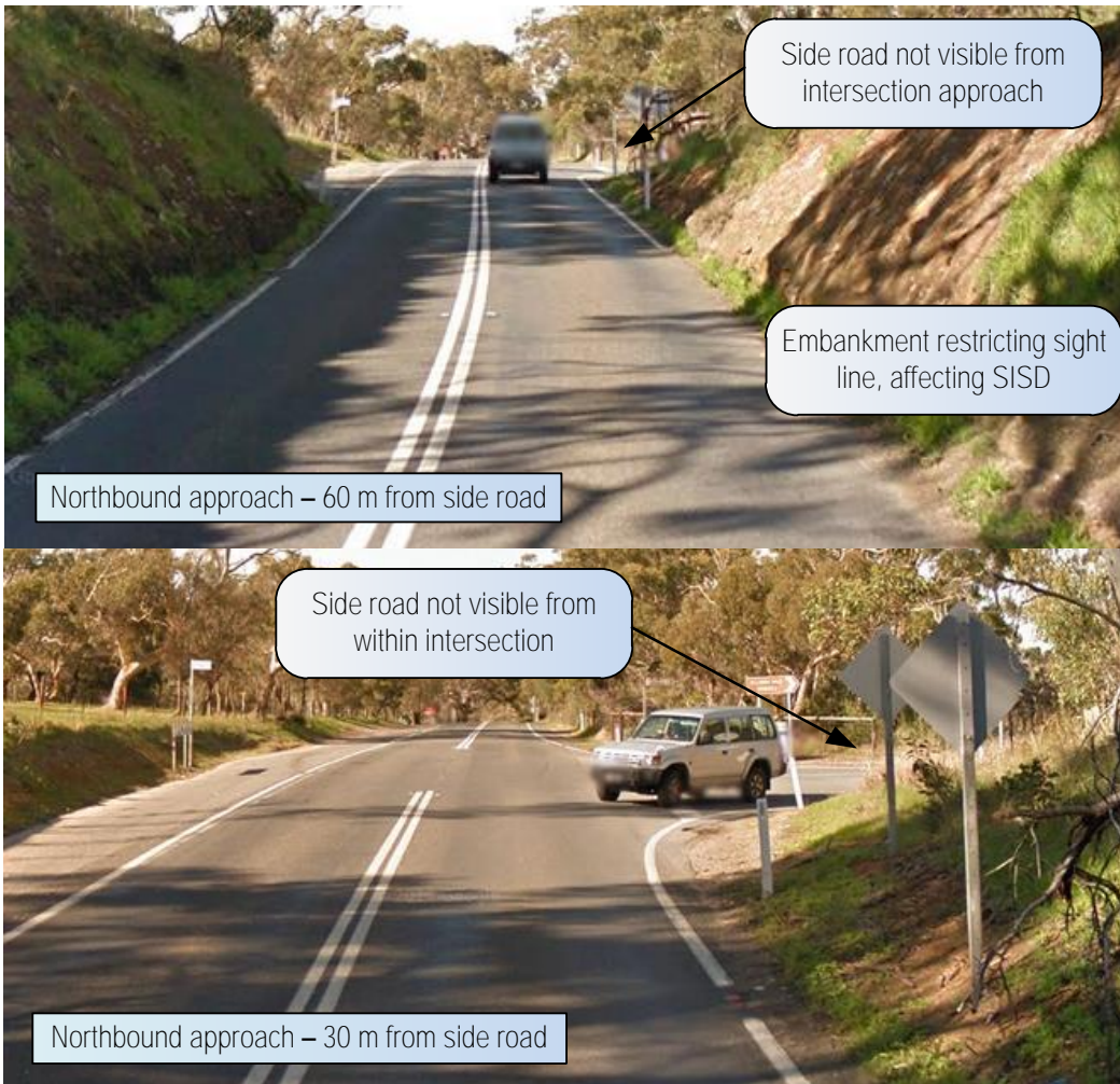
Figure 4.79: Rural – restricted safe intersection sight distance and visibility to side road from approach
