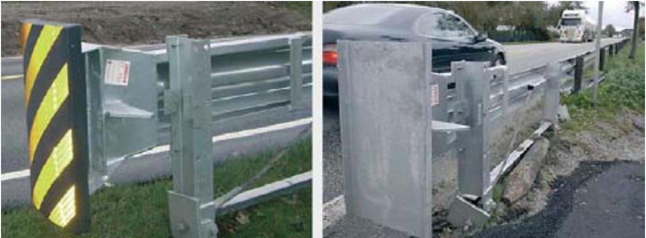
Figure 4.111: End terminal (ET2000) with and without cover
