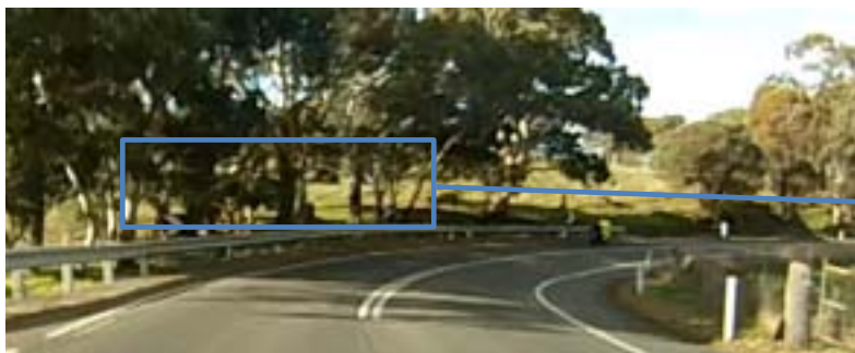
Figure 4.45: CAMs not conspicuous and hazard markers used
