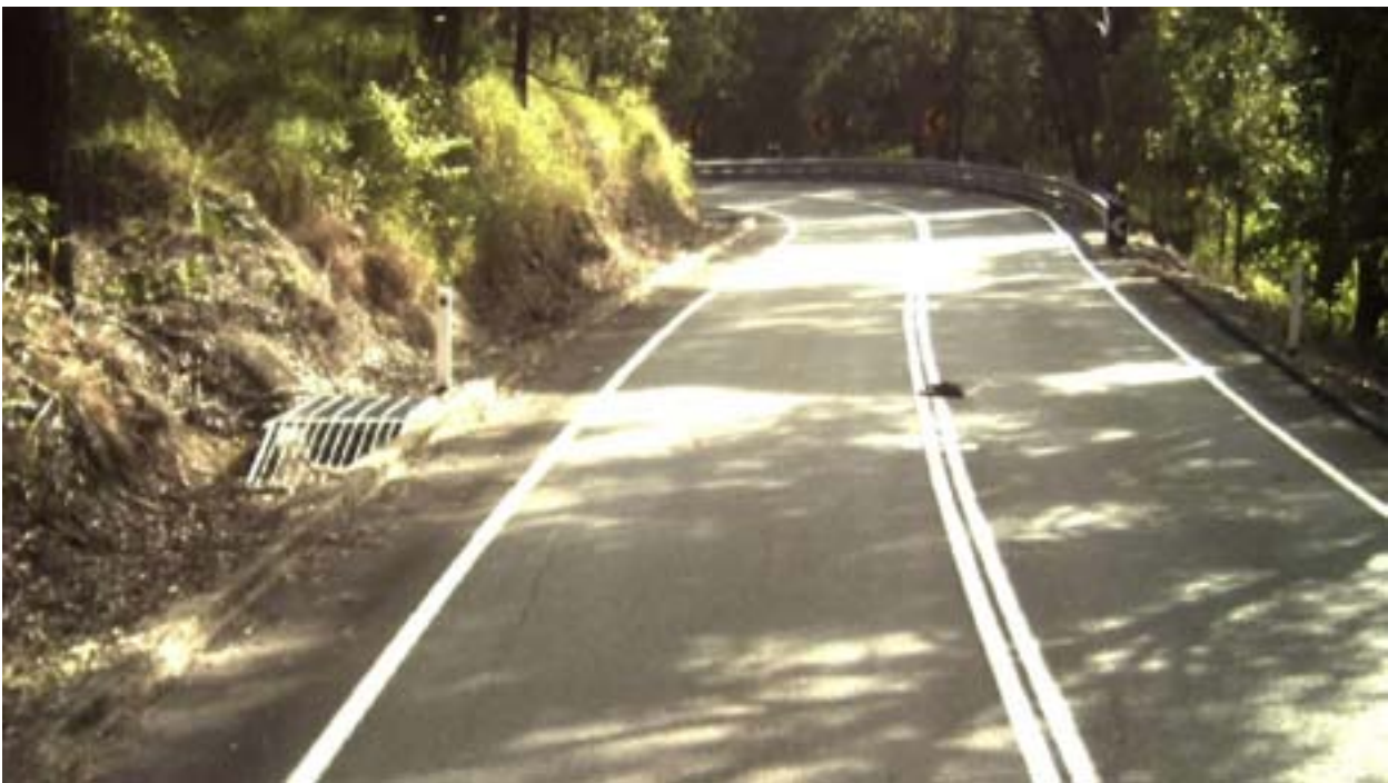
Figure 5.10: Traversable grate over perpendicular culvert face
