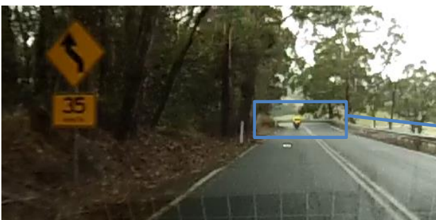
Figure 4.41: CAMs not provided on reverse compound curve with sharp curve warning and speed advisory plate
