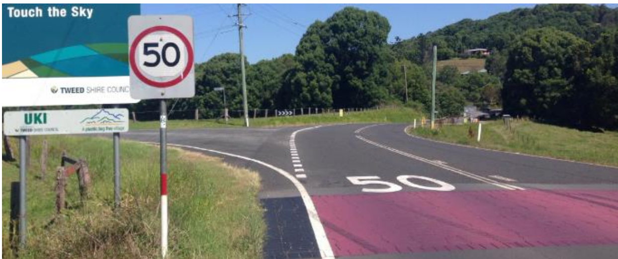
Figure 4.51: Painted pavers and pavement marking in braking and turning zone
